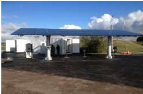
Hardware and software system integrators
